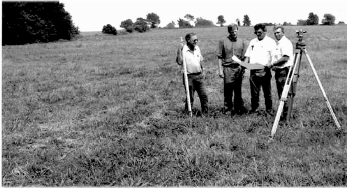
James Pinion (second from left) SCS team surveying site for JOMP.
