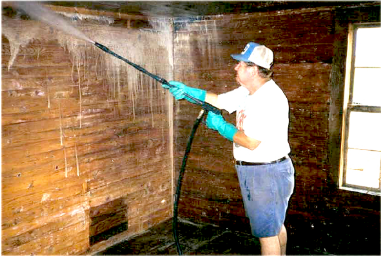
Curtis Cole cleaning the inside of the new Jesse Owens Memorial Park Birth Home Replica.
