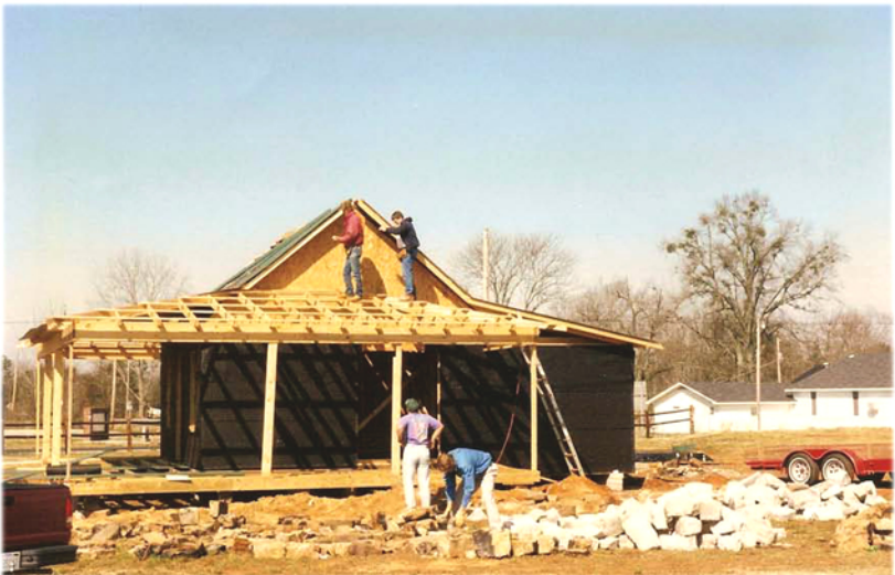
Adding a porch around house.
