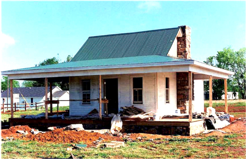
Stone chimney and fireplace completed.
