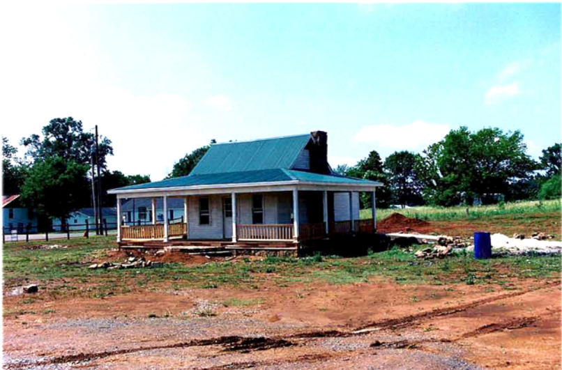
Porch rails installed.
