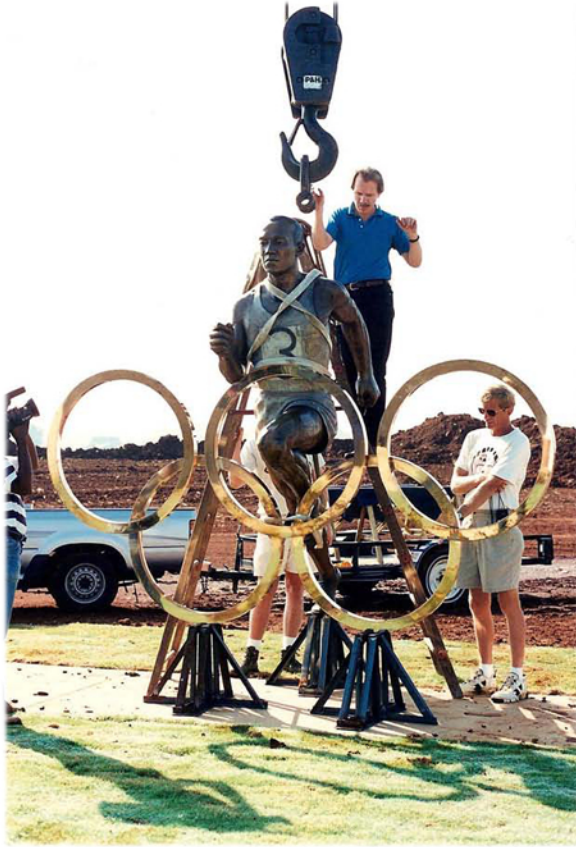
Strapping the statue securely to be hoisted onto its permanent base.
