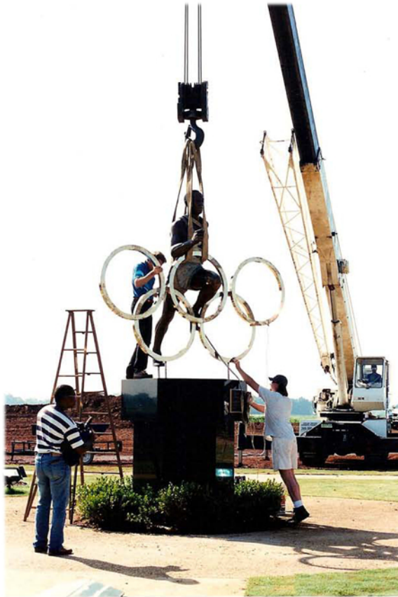
Statue being permanently anchored on its base.
