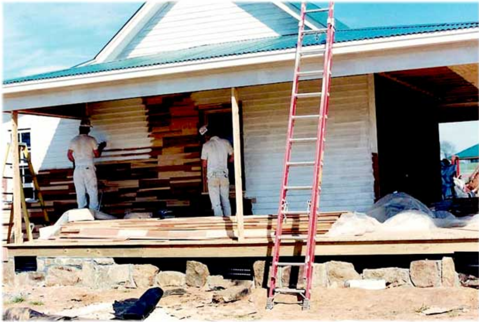
Cedar siding being painted on new Welcome Center.
