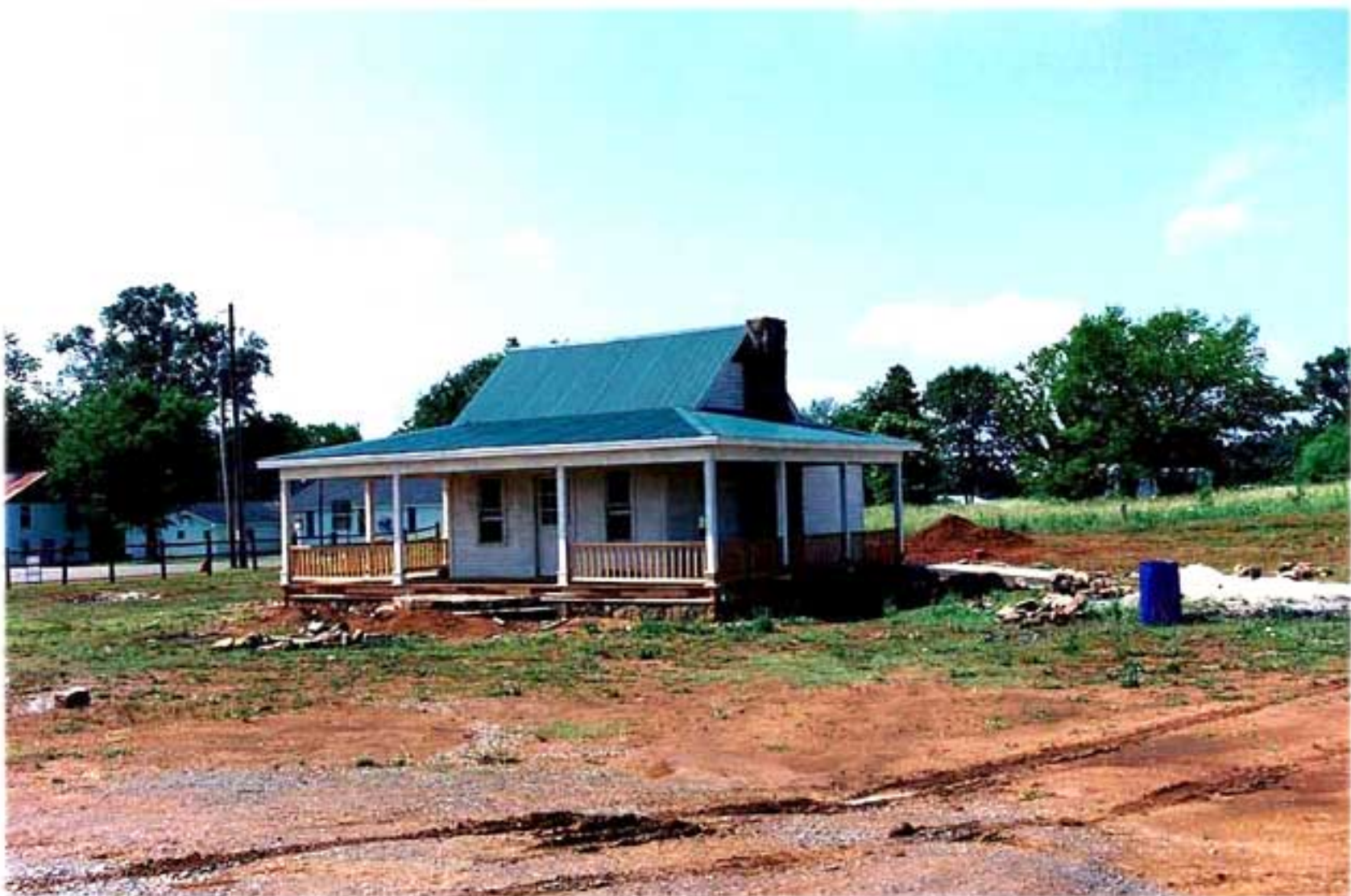
Porch rails installed.
