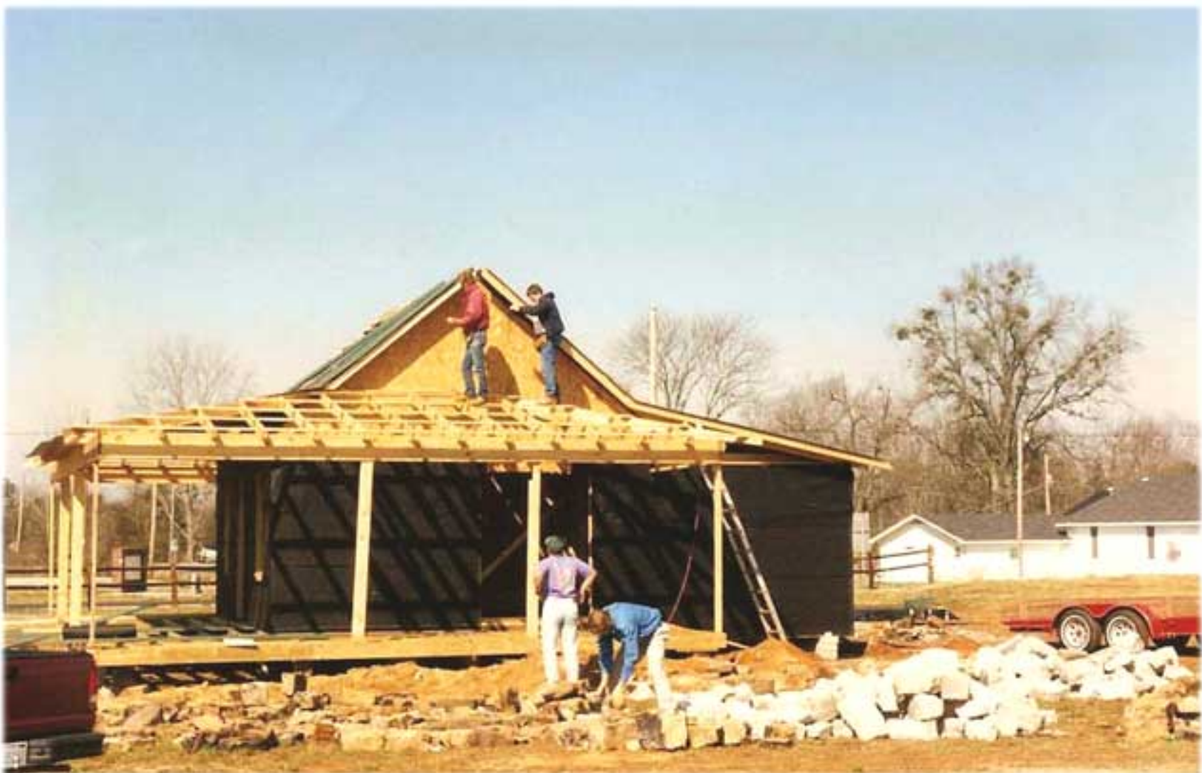
Adding a porch around house.
