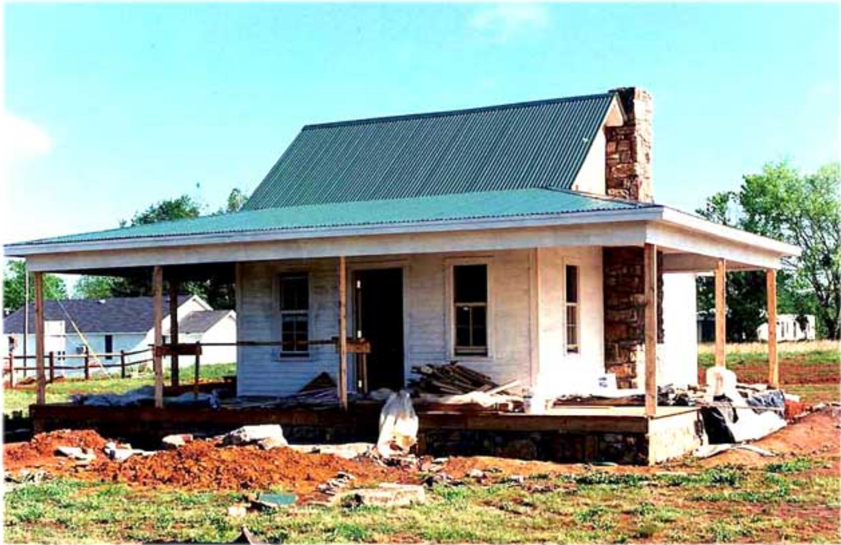
Stone chimney and fireplace completed.
