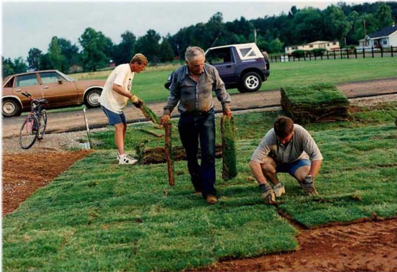
Laying sod at Visitor's Center. Left to Right: James Pinion, Don Rojem & Kenneth Lambert
