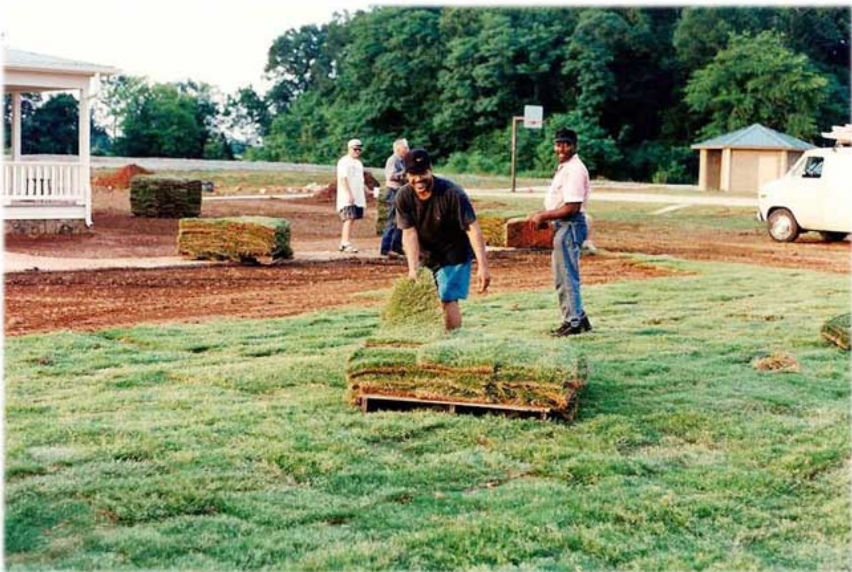
Bermuda sod being laid around the Welcome Center.
