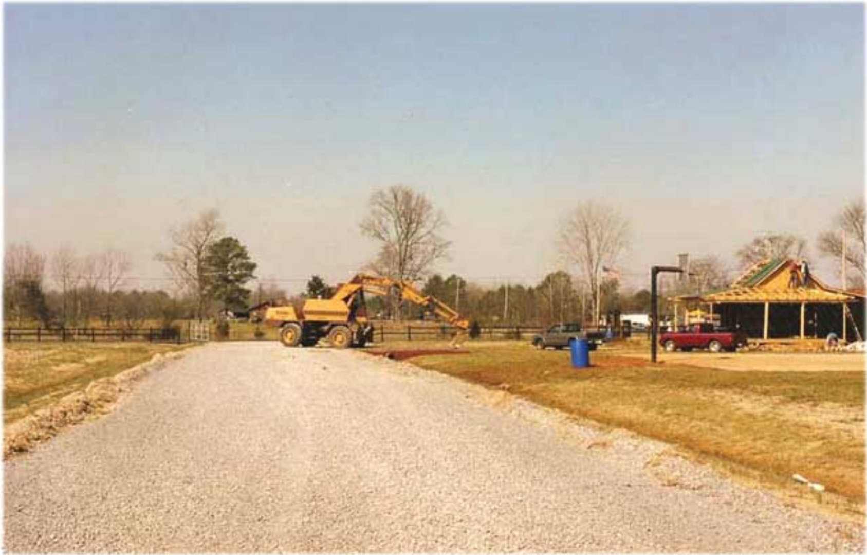
Working on Visitor's Center and culvert into entrance. Barrett Shelton, Decatur Daily gave $27,000 to restore the house.
